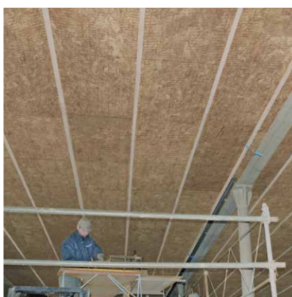
Solai o travature
